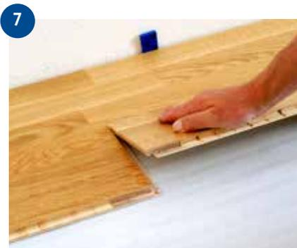
7 Fold the panel down in a single action movement with a slight press to the short end of the previous panel. During the fold down, make sure the panels are tight against each other.
