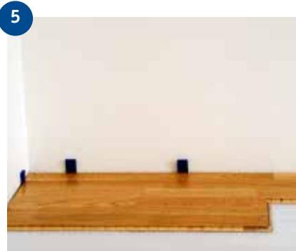
5 First plank, second row. Start with the rest of the cut board from the first row. Ensure that all the short end joints are staggered from the short end joints of the other row by at least 50 cm.
