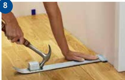
Tap in the sawn board using the pull bar. If the final row of boards has not been cut, the tongue must be sawn off in order to keep an expansion gap. If installing T & G place spacers along the final row of boards too. Now that the floor has been installed, skirtings and any joining strips can be fitted but don't forget to remove all the spacers.
