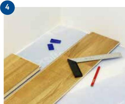
4 At the end of the row, turn the last board so that it lies tongue to tongue. Push the short end tightly against the wall. Mark where to cut with a pencil 8-10 mm from the previous board's short end to give you an expansion gap when the board is tapped into place.
