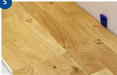
Viva Ultraloc, which has a middle layer of HDF, is tapped together along the long side first. Then tap the short ends together. For other Ultraloc boards the short ends are tapped together first, followed by the long side, starting with the free end. The long side groove must be placed against the tongue for this.
