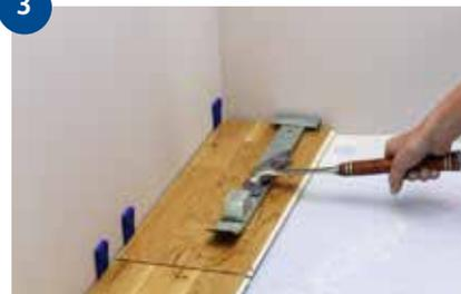
Cut the board where you marked. Angle it into place and tap it in with the pull bar. Place a spacer between the short end and the wall.
