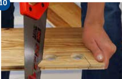
If the long side of the board meets a pipe: Drill a hole with a diameter min. 16 mm greater than the pipe diameter to give an expansion gap around the pipe. Mark with a pencil where to saw. Saw off the bit which will fit behind the pipes, closest to the wall. Cut at an angle as shown in the picture. If the pipes are located along the short side of the floor, cut the board at a 90° angle straight through the holes.
