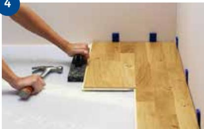
Start the second row with the rest of the cut board. Ensure that all the short end joints are staggered from the short end joints of the other row by at least 50 cm for boards longer than 1250 and at least 30 cm for boards shorter or equal to 1250 (e.g. Viva).
