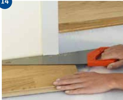
Doorframes can be removed and moved up, but it is usually easier to saw them off. Use a loose floorboard as a height template and saw the frame with a fine-toothed saw. Push the floor under the frame. Ensure that the floor is not wedged between the subfloor and the frame.
