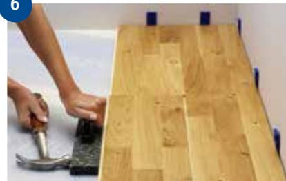
Continue installing the subsequent rows in the same way until you reach the final row. Always start a new row with the rest of the cut board from the end of the previous row. Use a hammer and Tarkett's installation tools: tapping block and pull bar. Do not tap the boards together with excessive force. This and/or using the wrong tools will cause chipped edges.
