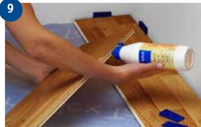
Boards with Tongue & Groove should be point bonded. That is a generous line of glue, about 10 cm long, placed in the groove with a half-meter intervals. The groove in the short end should be glued all the way.
