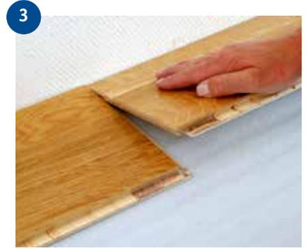
3 Second plank, first row. Place it gently and tight to the short end of the first one. Fold the panel down in a single action movement. During the fold down, make sure the panels are tight against each other. Afterwards press or slightly knock at the short end just installed.
