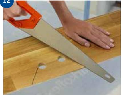
If the long side of the board meets a pipe: Drill a hole with a diameter min. 16 mm greater than the pipe diameter to give an expansion gap around the pipe. Mark with a pencil where to saw. Saw off the bit which will fit behind the pipes, closest to the wall. Cut at an angle as shown in the picture. If the pipes are located along the short side of the floor, cut the board at a 90° angle straight through the holes.
