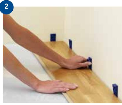
2 First row. Remember that the floorboards should preferably run along the length of the room. Start in a left-hand corner with the groove side against the wall and work towards the right. The next board is angled down into the short end of the previous board so that it slides into place. Press spacers between the floor and the wall to create an expansion gap of 8-10 mm, after approx. 3 rows is recommended.
