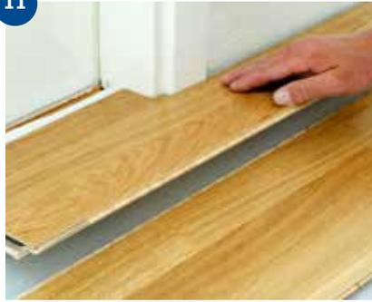
Then tap the board sideways with a pull bar. Finish by placing spacers in the expansion gap between floor and wall. Now that the floor has been installed, skirtings and any joining strips can be fitted but don't forget to remove all the spacers.
