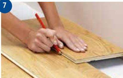
Final row: When you get to the final row, it is possible that the boards will not fit width wise. In this case, place the final board with the tongue facing the wall, on top of and edge to edge with the last-but-one board. Place a spare bit of board on top and measure the gap by running the bit of board along the wall and marking with a pencil where to cut the final board.
