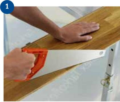
1 Before installing the first row, the part of the groove profile which sticks out must be cut off.
