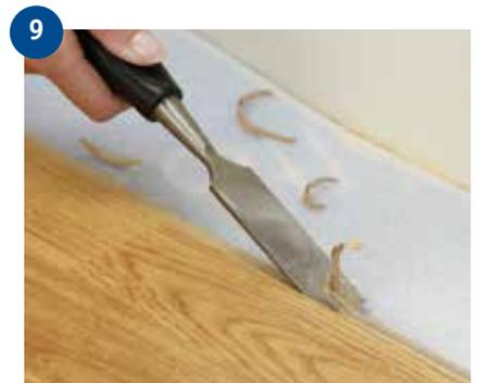
9 If there is no room to fold down the last board, it can be slide in from the side instead. In order to do this, the tongue of the board in the previous row has to be made level. Use a chisel to shave off the part of the tongue which raises like a bump along the top of the outside edge.
