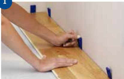
First row. Remember that the floorboards should preferably run along the length of the room. Start in a left-hand corner with the groove side against the wall and work towards the right. If the wall isn't straight, cut lengthwise. Place the tapping block against the short end of the board and tap the boards together with a hammer. Press spacers between the floor and the wall to create an expansion gap of 8-10 mm.
