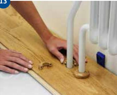
Tap the board in position, glue the loose piece in place, fit a spacer against the wall and cover with pipe collars.
