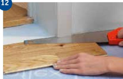
Doorframes can be removed and moved up, but it is usually easier to saw them off. Use a loose floorboard as a height template and saw the frame with a fine-toothed saw. Push the floor under the frame. Ensure that the floor is not wedged between the subfloor and the frame.
