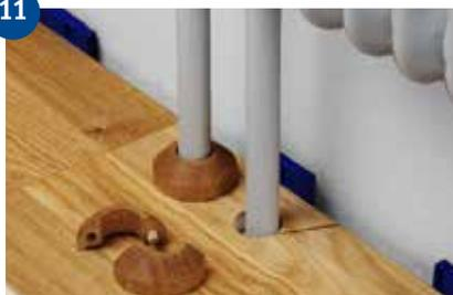
Tap the board in position, glue the loose piece in place, fit a spacer against the wall and cover with pipe collars.
